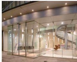
NT Building (entrance)
