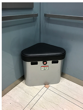
NT Building Emergency supplies installed in elevators
