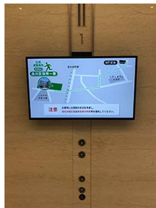
NT Building Digital signage
