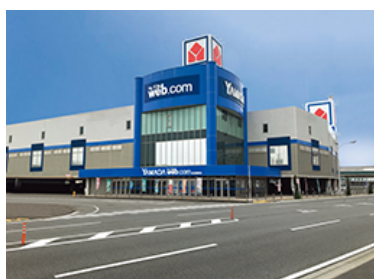
C-05 YAMADA web.com Matsuyama Toiyacho (Rooftop Solar Panel)
